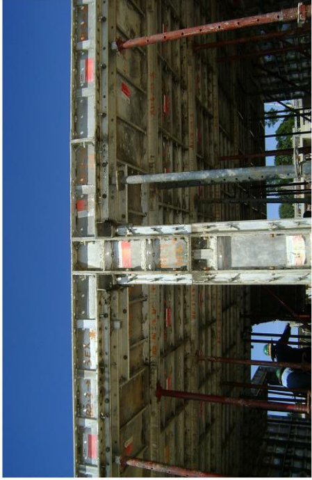
FIRST FLOOR SLAB FORM WORK (200MM R.C. THICK SLAB)
