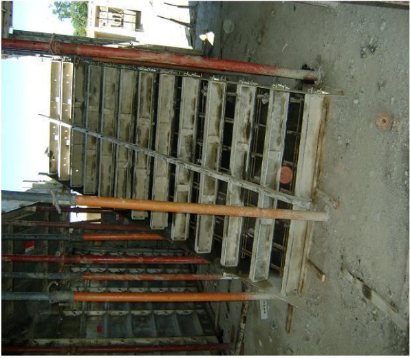
STAIRCASE FORMWORK
