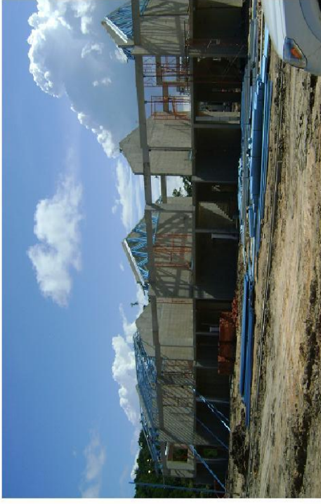
PHASE 3 & 4 AND 5 & 6 TANAH JAMBU TERRACE HOUSING. THE USE OF ALUMINIUM FORM WORK FOR 1,098 UNITS OF TERRACE LINK HOUSES. AVERAGE COMPLETION OF 60 TO 75 STRUCTURAL FRAME PER MONTH.
