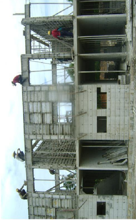
PHASE 3 & 4 AND 5 & 6 TANAH JAMBU TERRACE HOUSING. THE USE OF ALUMINIUM FORM WORK FOR 1,098 UNITS OF TERRACE LINK HOUSES. AVERAGE COMPLETION OF 60 TO 75 STRUCTURAL FRAME PER MONTH.
